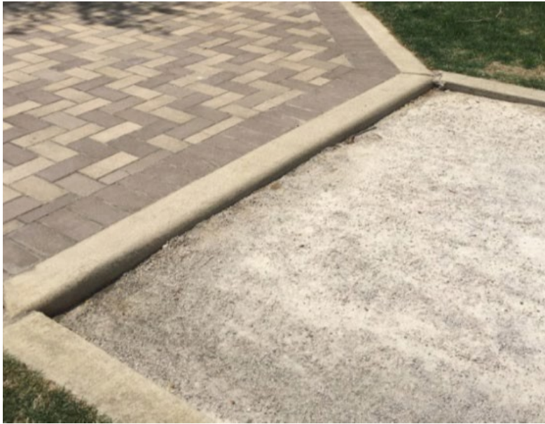
Picture 3: Level Changes at Dissimilar Materials
