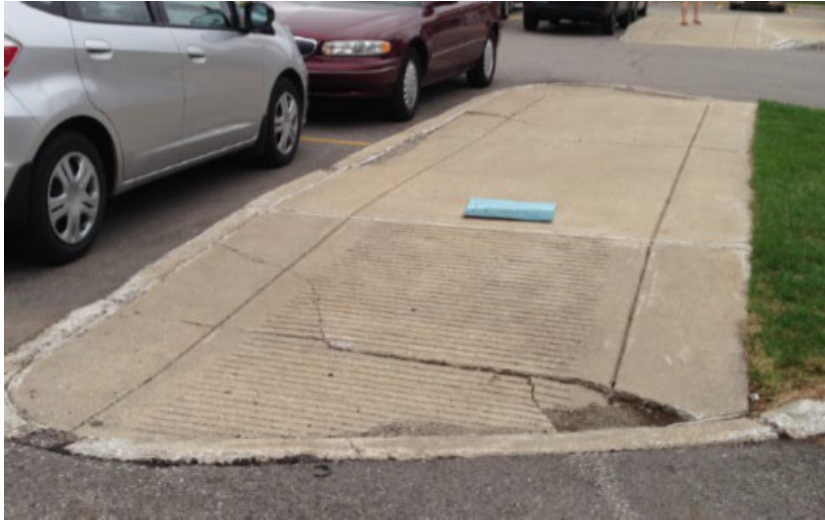
Picture 1: Curb Ramps
